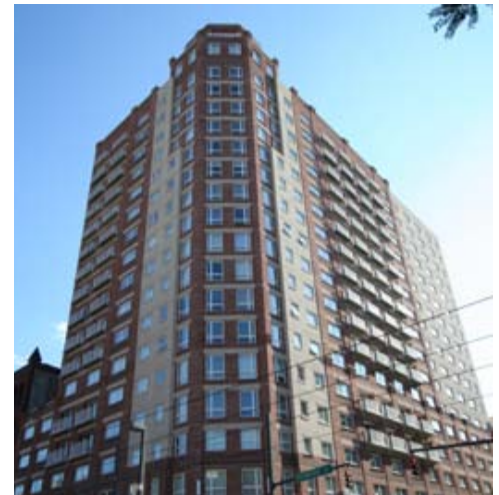
Centerpoint Tower - Baltimore, MD
