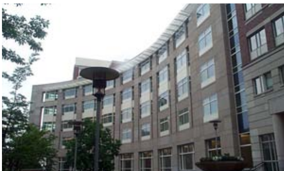
UMB Health Science Facility II
