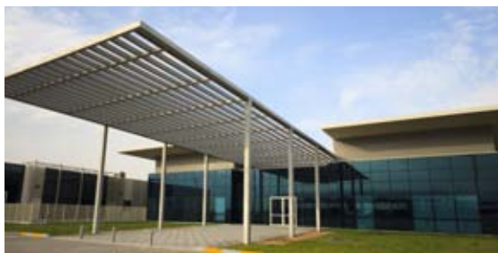
Custodian Care Facility - Abu Dhabi, UAE
