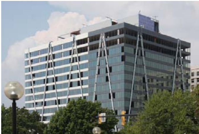
Hoffman Center Building 1 - Alexandria, VA
